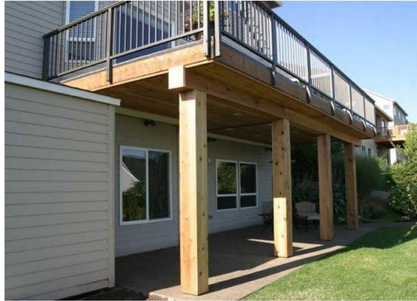
Figure 5: Example of pressure-treated deck
