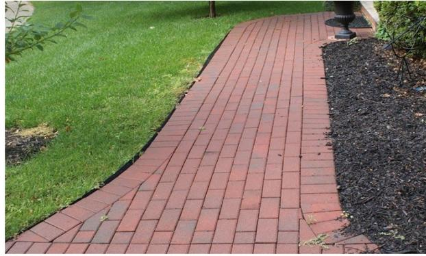
Figure 4: Example of Paver Walkway
